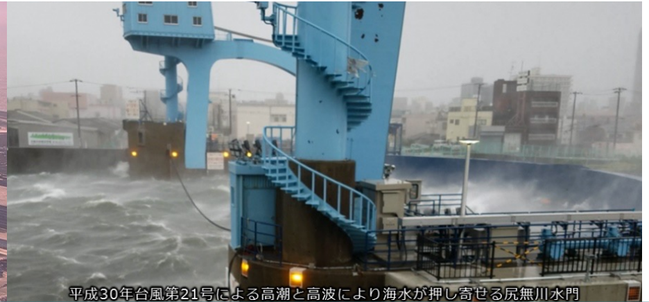
Seawater rushing to the sluice gate due to storm surge and high waves in Osaka.
