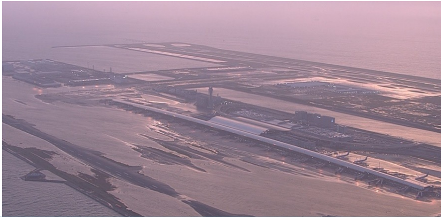
Inundation of airport facilities (Kansai International Airport)
